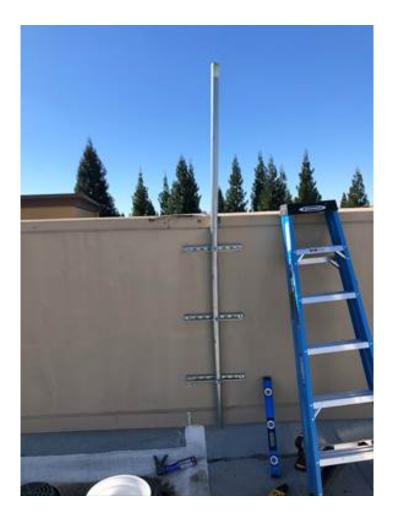
Cut All-Strut pieces to length. Three pieces ensure a robust connection to the parapet that can sustain gusty winds.
